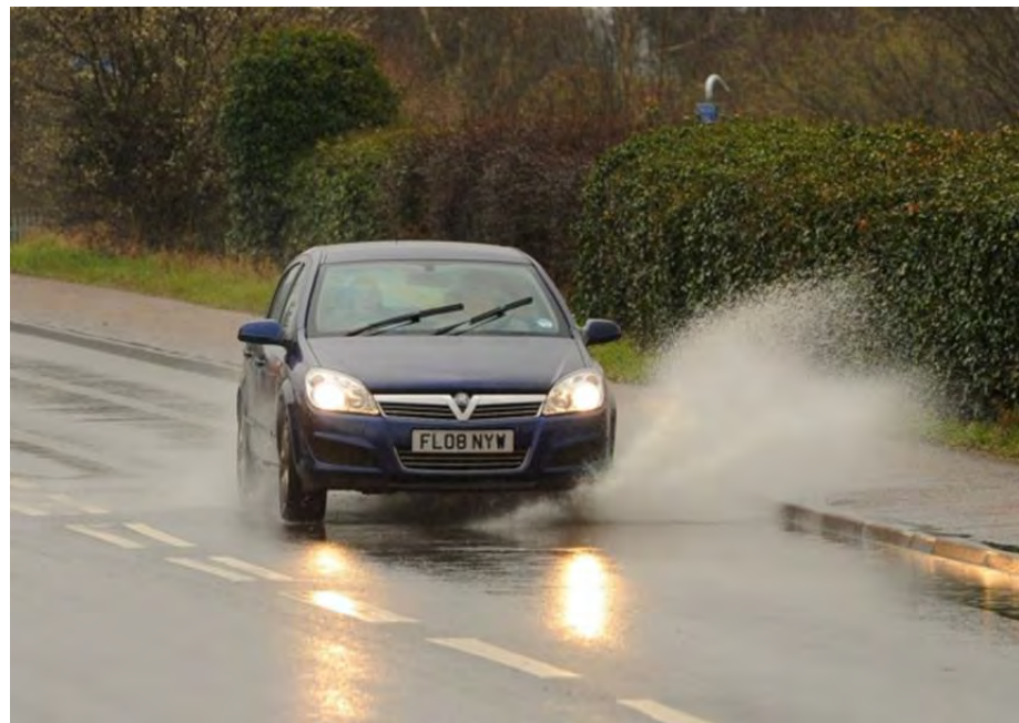
Figure: 1.1 Accumulation of puddles on highway road during rain time.
