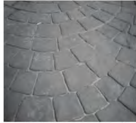
b) Pavement road surface
