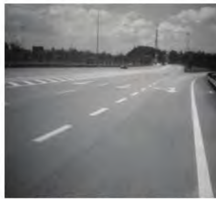
a) Highway road surface
