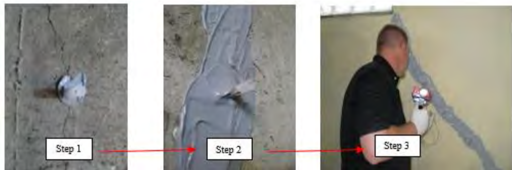
Figure 2.5 : Step of injecting polyurethane foam (Eastern, 2012)
