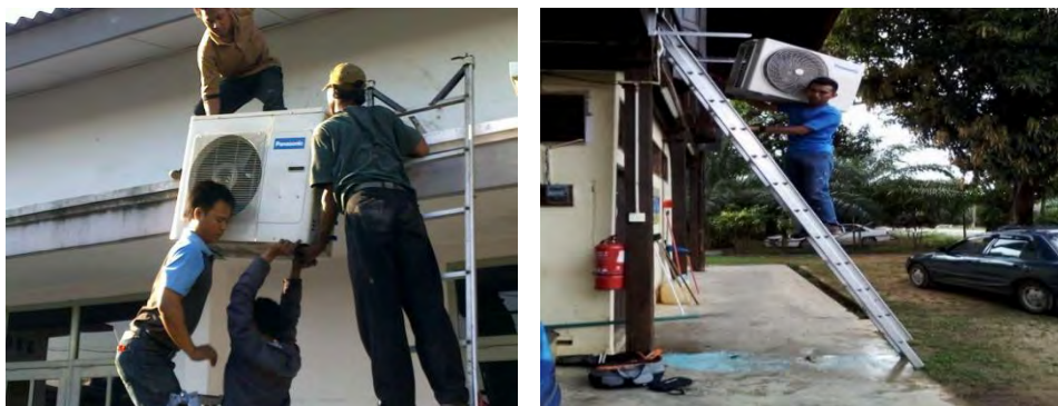
Figure 1.1 Man power to lifting outdoor unit
