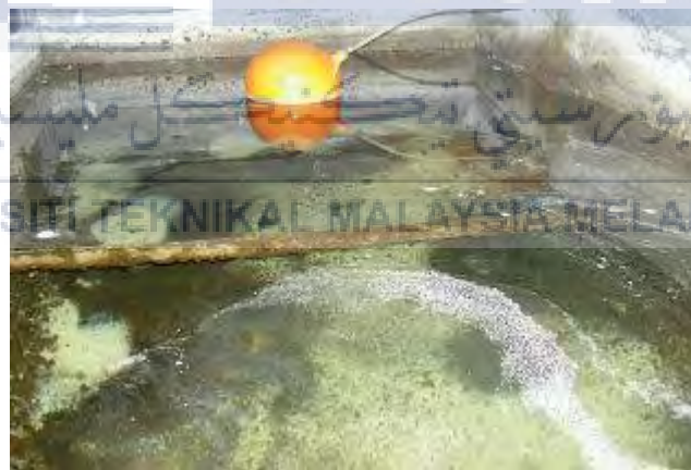
Figure 2.1: Water tank that has been infected with Legionella [17].
