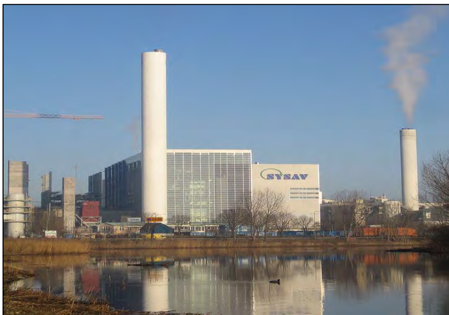
Figure 2.1: SYSAV incineration plant in Malmö, Sweden, capable of handling 25 metric tons (28 short tons) per hour of household waste.
