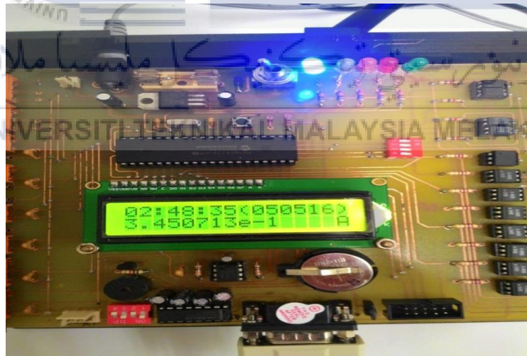
Figure 4.7: Undervoltage condition displayed
