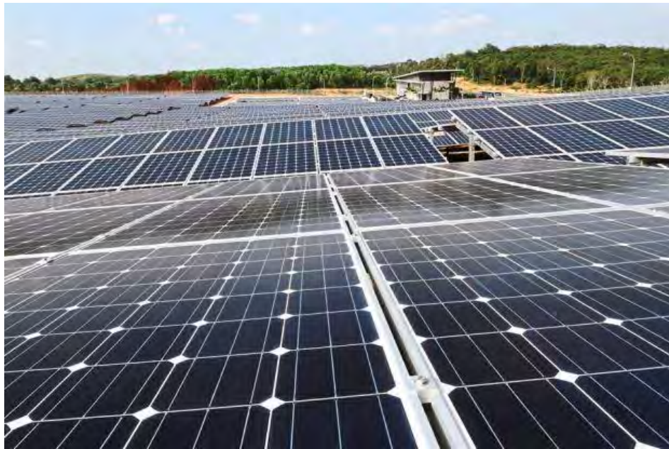
Figure 2.4: Grid Connected Solar Farm in Melaka, Malaysia
