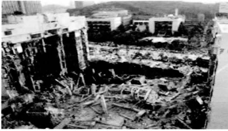
Figure 2.2: Sampoong Department Store collapse in South Korea (Anonymous n.d.)
