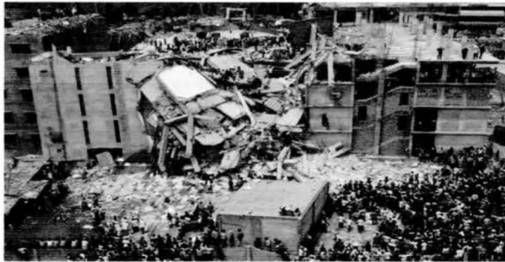
Figure 2.1: Rana Plaza collapse in Bangladesh (Schwier 2013)
