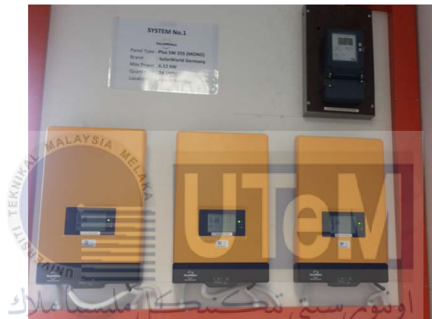
Figure 3.3: PV inverter model of SMA Sunny Boy 2000HF
