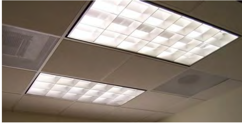
Figure 3.4: Recessed parabolic fluorescent (T12) with 2" fixture [33]
