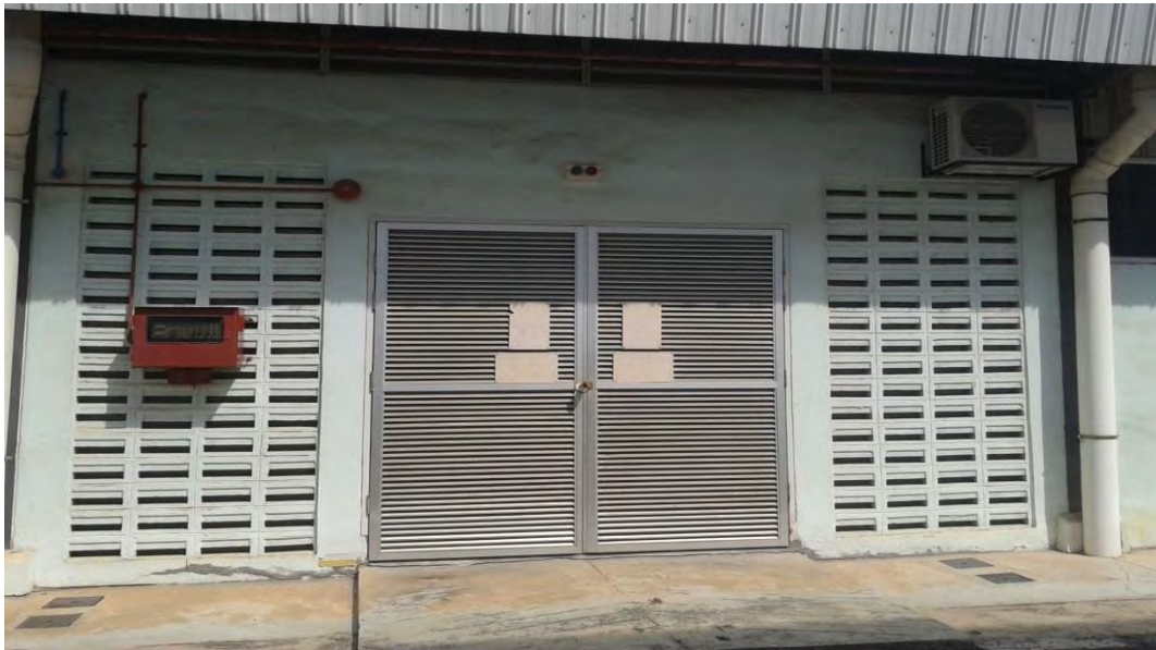
Appendix C: Server room Factory 1
