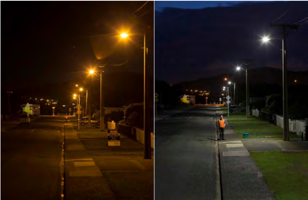
Figure 2.8 Smart street lighting
