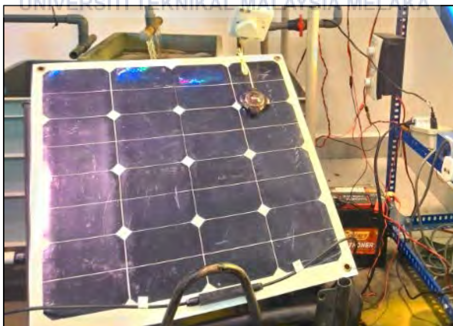
Figure 3.8: The complete model of installing flexible solar panel
