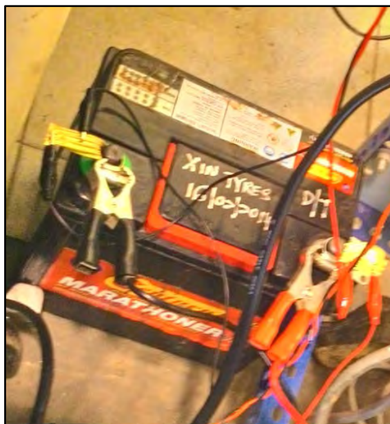
Figure 3.12: Battery that supply power to the system
