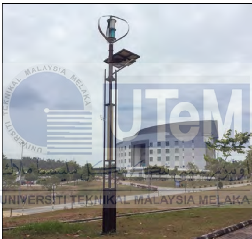
Figure 2.10: Hybrid PV-Wind System installed at FKE courtesy of [9]
