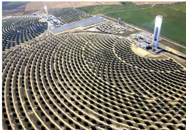
Figure 1.4: Solar thermal electric facility in Seville, Spain (Caldés et al. , 2009)
