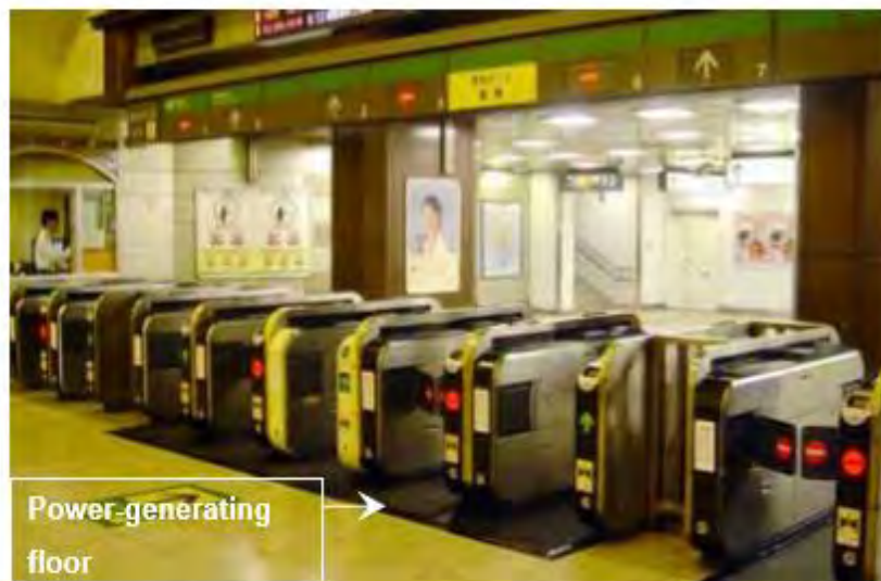
Figure 4 “Power-generating floor” was installed at the ticket gates of train stations in Tokyo
