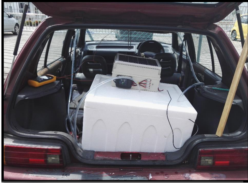
Figure 32 Picture of Serpentine Pattern of Copper Tube Installed at the Ceiling of Car with Connection the Hydronic Cooling System
