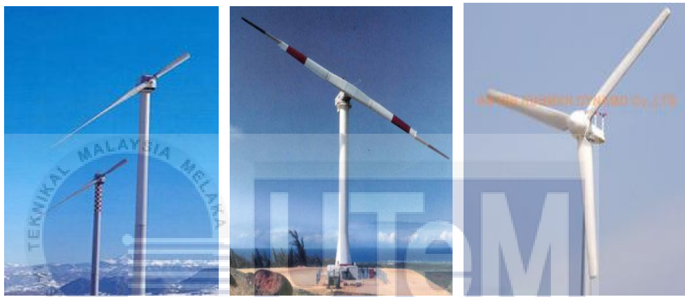
Figure 3.3 Structure of single, two and three horizontal wind turbine blades.
