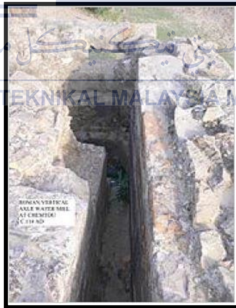
Figure 2.1: Roman turbine mill at Chemtou, Tunisia. The tangential water inflow of the millrace made the submerged horizontal when in the shaft turn like a true turbine. (Wilson, 1995)
