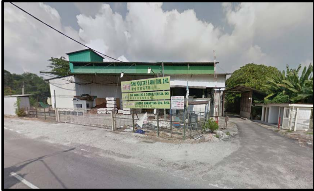
Figure 1.1: SHH Poultry Farm Sdn Bhd building
