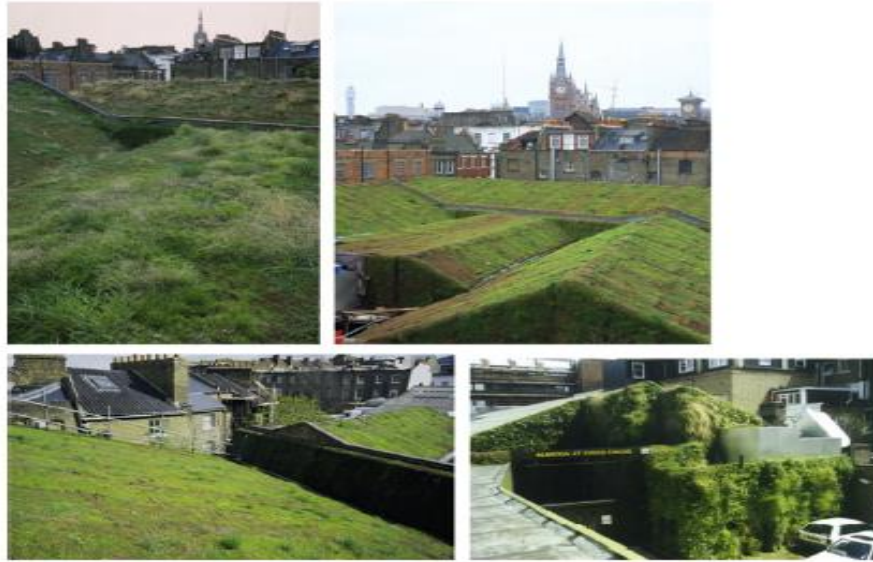
Figure 2.7: Building greenery as acoustic insulation. Almeida Theatre. London (Perez et al., 2016).
