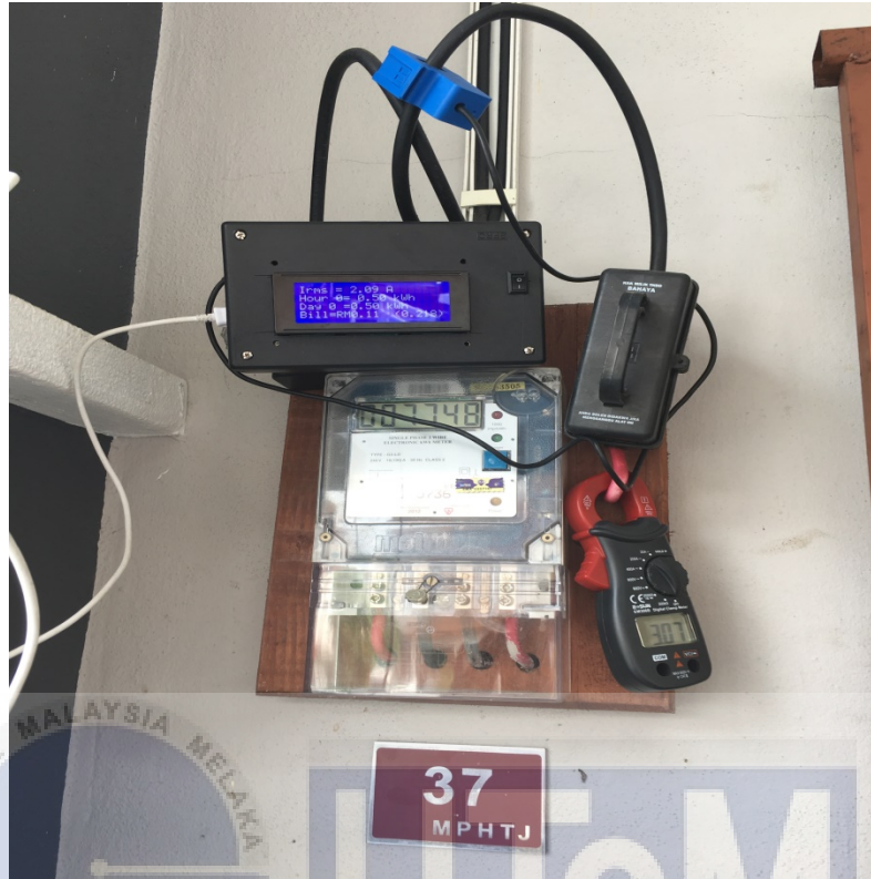
Figure 4.3 : The installation of the Smart Domestic Electricity Monitoring System
