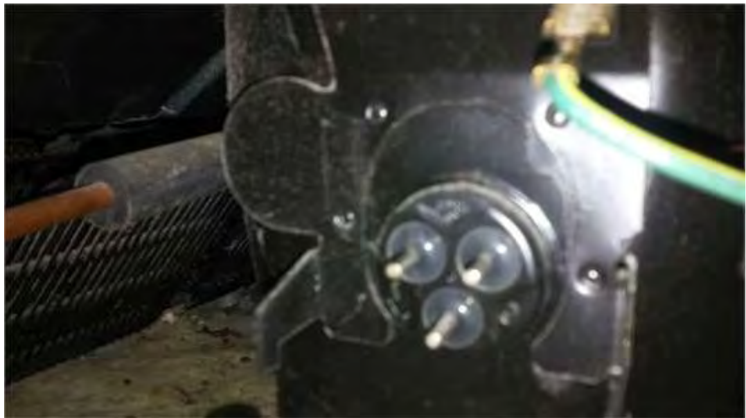
Figure 1.3: Compressor for refrigerator that does not have terminal markings (Brand: Embraco, Model: EGY90HLP)
