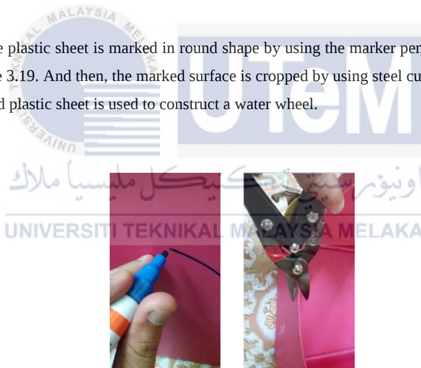
Figure 3.20: Marking and Cutting The Plastic Sheet
