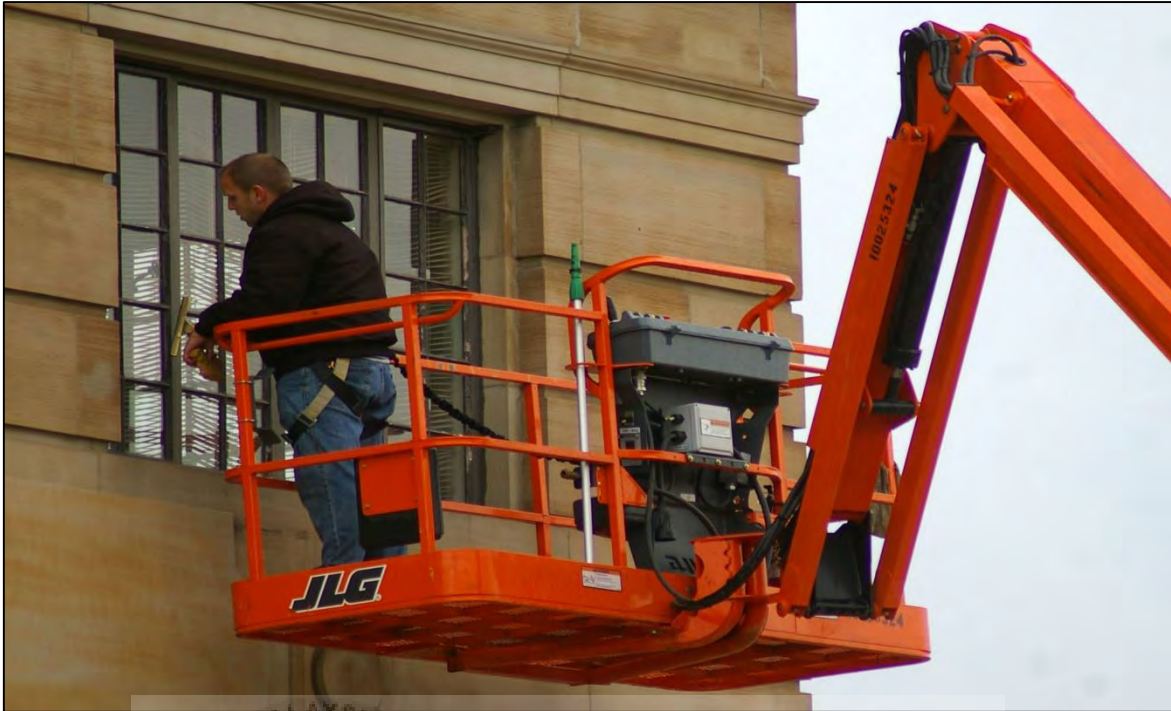
Figure 1.4: Workers using crane for their job
