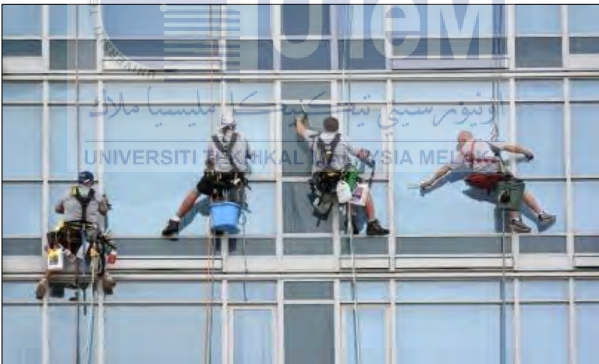
Figure 1.2: Worker cleaning the window using Bosun's chair
