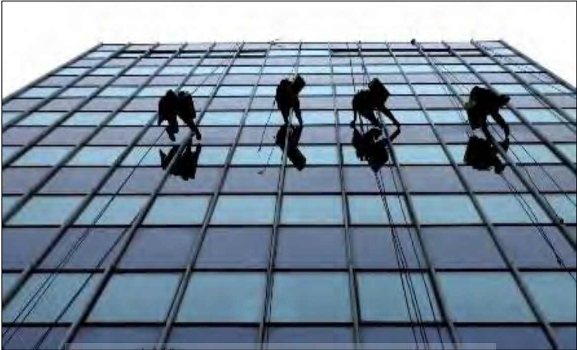
Figure 1.1: Workers complete their task using Bosun's chair
