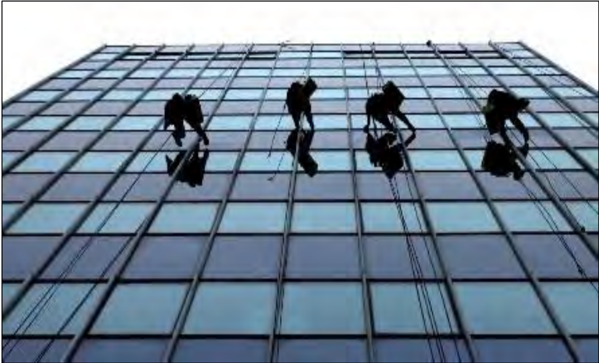
Figure 1.1: Workers complete their task using Bosun's chair
