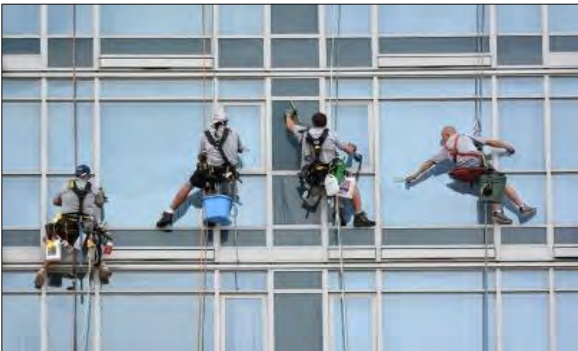
Figure 1.2: Worker cleaning the window using Bosun's chair
