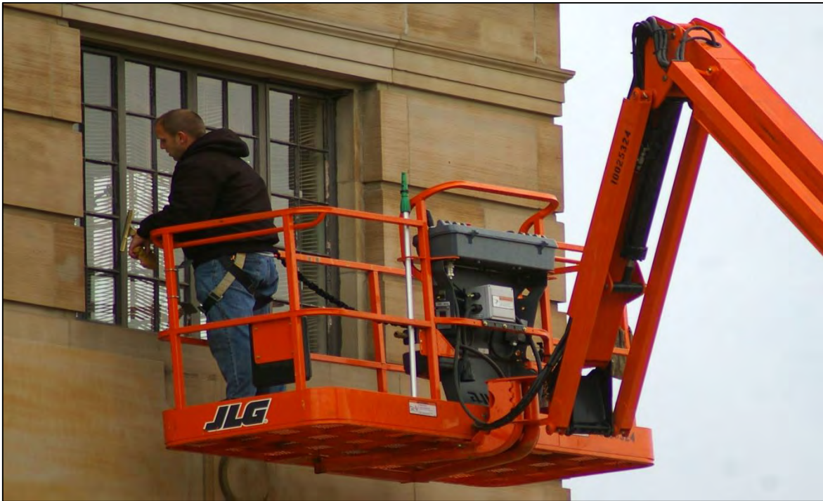
Figure 1.4: Workers using crane for their job
