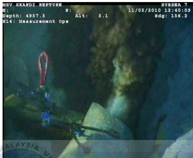
Figure 1.1: Broken 21” oil pipe 5000’ down in the Gulf of Mexico taken by ROV [7]
