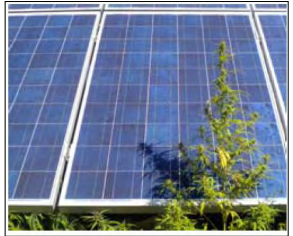
Figure 2.3: The Surrounding Plant and Guano Shading Phenomenon
