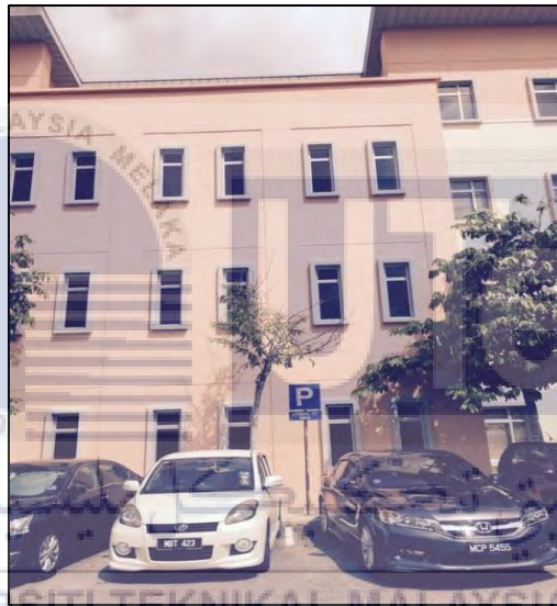
Figure 4.12: The 15m FKE building
