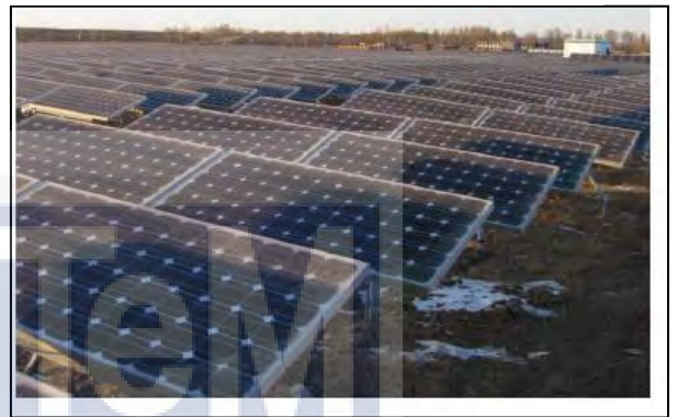
Figure 2.4: Front Row Shading Phenomenon
