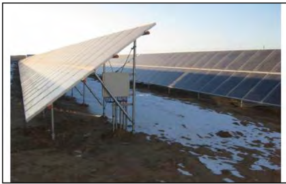
Figure 2.4: Front Row Shading Phenomenon
