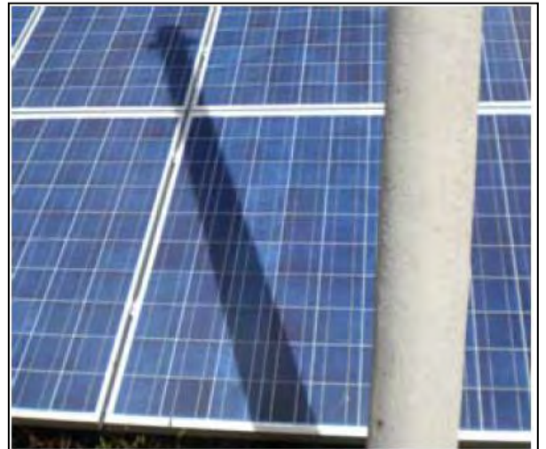
Figure 2.5: The Nearby Power Distribution Room and Wire Pole Shading Phenomenon
