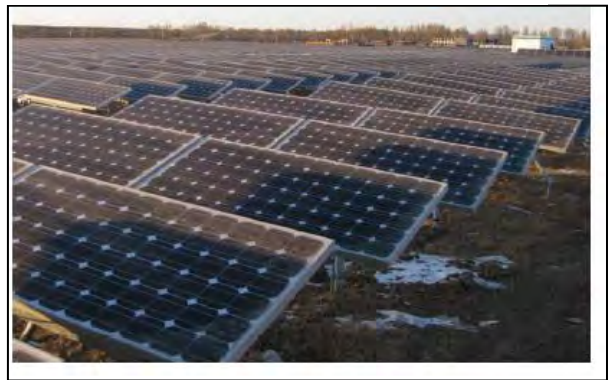
Figure 2.4: Front Row Shading Phenomenon
