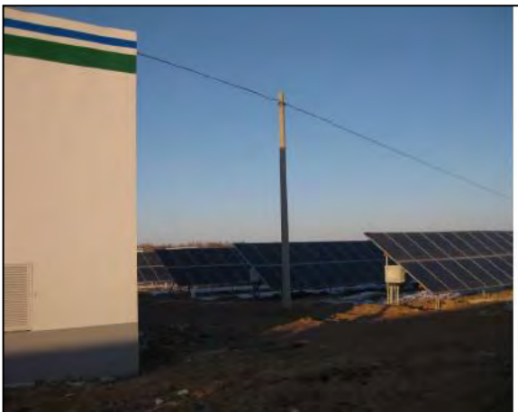
Figure 2.5: The Nearby Power Distribution Room and Wire Pole Shading Phenomenon
