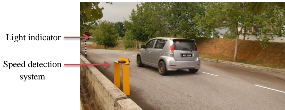
Figure 4.3: The placement of the speed warning system
