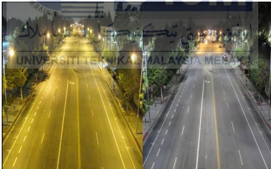
Figure 2.2: The different lighting between HPSV lamp and LED lamp [16]
