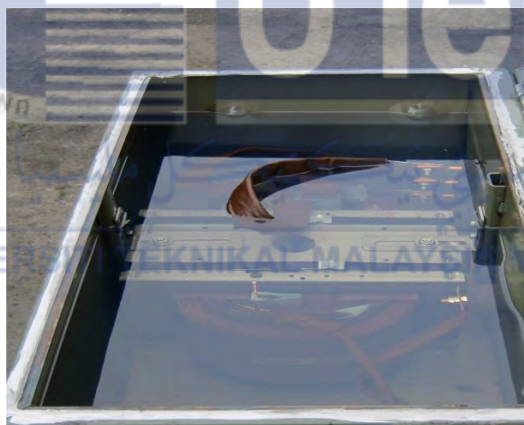
Figure 2.2: Insulating oil in an electrical power transformer [13]
