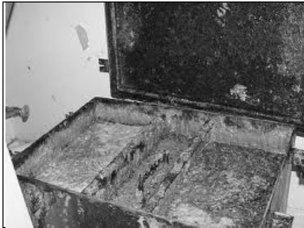
Figure 4: Example of overflow grease trap (Source: Lakasa, 2006).
