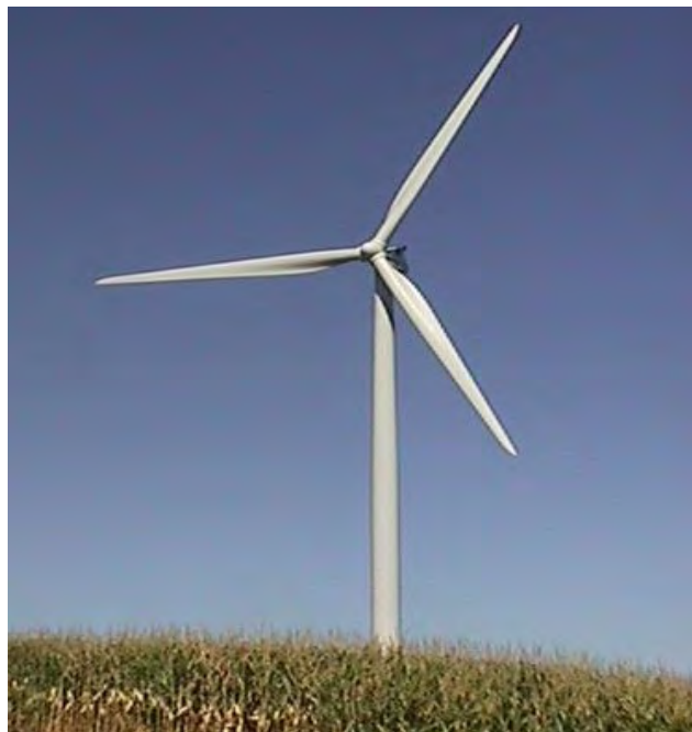
Figure 2.3: Horizontal Axis Wind Turbine (HAWT)
