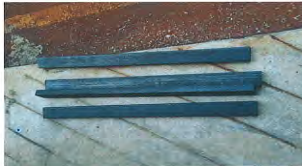
Figure 3.4: Material already cut
