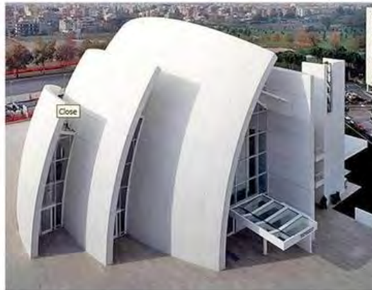
Figure 1.2: Jubilee Church of Rome, Exterior made from Italcementi Concrete Containing TiO 2 (Hashimoto et al; 2005)
