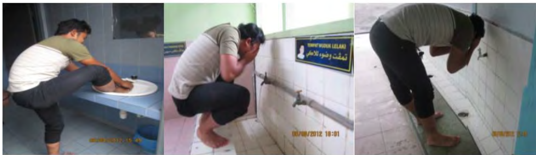
Figure 1.1: The variation of ablution station.
