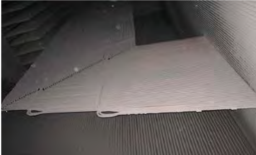
Figure 2.3 : Super-heater tubes in boiler (Chong, Ahmad, & Purbolaksono, 2002)
