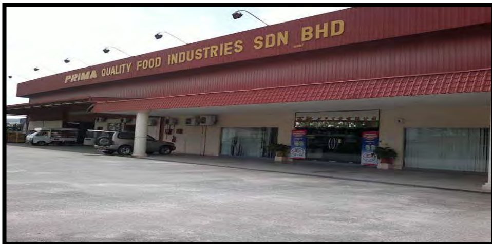
Figure 1.1: Front building of Prima Quality Food Industries Sdn Bhd
