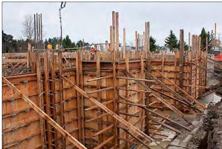
Figure 1.1: Reinforced Cement Shear Wall formwork system (plywood)
