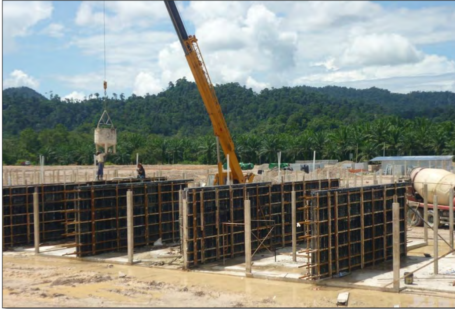
Figure 1.4: RC Shear wall formwork system (Polymer)
