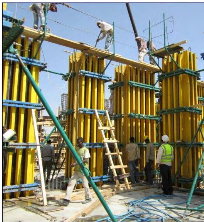
Figure 1.3: RC columns formwork system (Steel)
