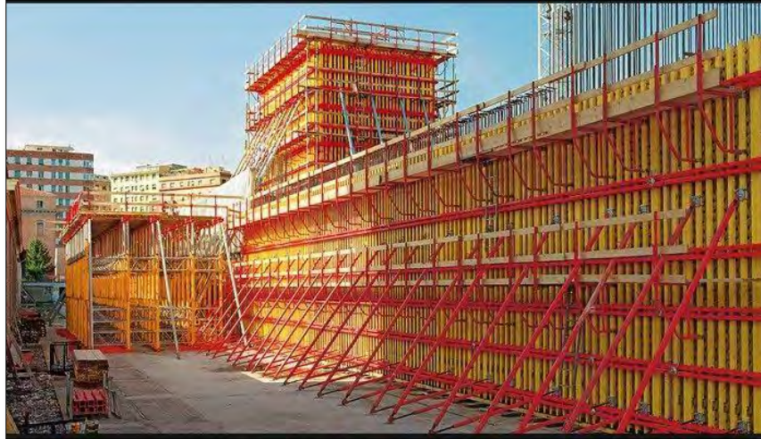
Figure 1.2: RC Shear wall formwork system (Steel)
