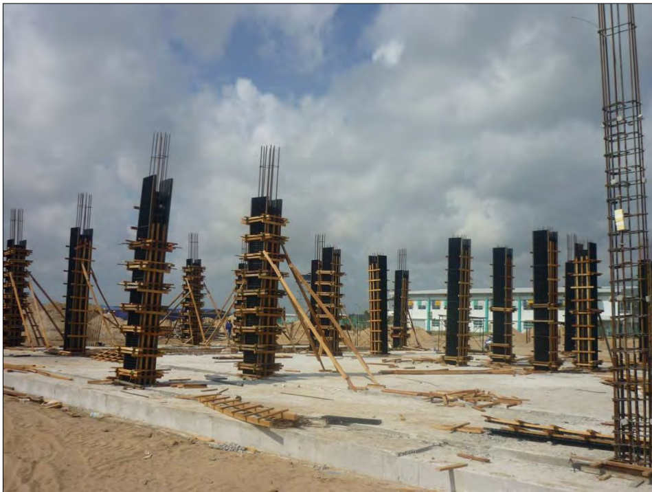
Figure 1.5: RC Columns Formwork System (Polymer)
