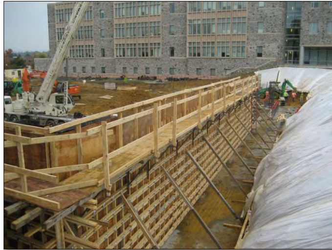
Figure 1.0: Ground beam formwork system (plywood)
