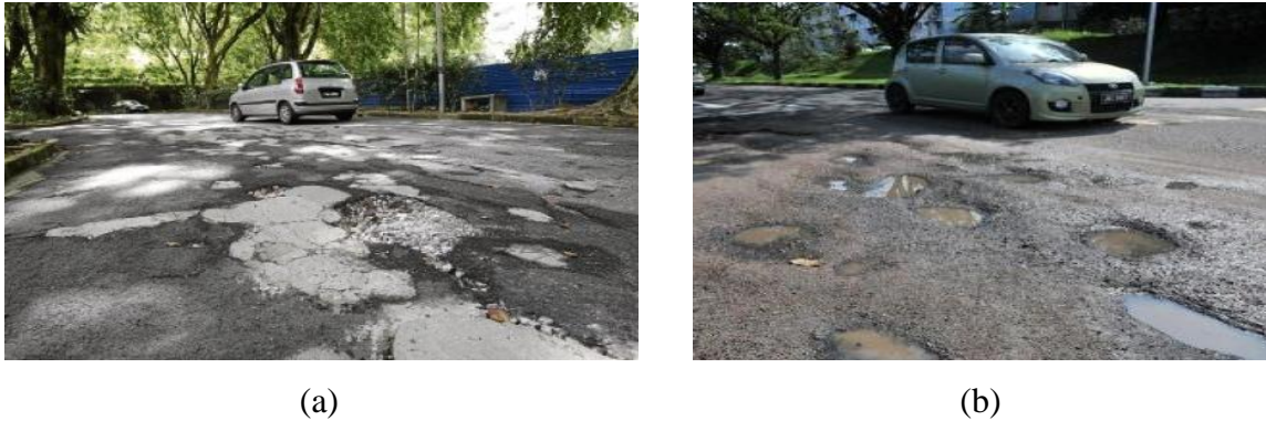
Figure 1.1: (a) Bad road quality in Malaysia [19] and (b) Pothole on the road surface in Malaysia [18]
