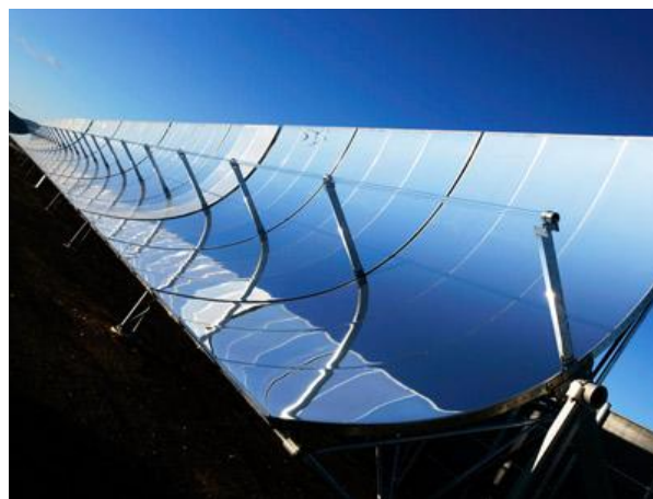
Figure 2.3: Parabolic trough
