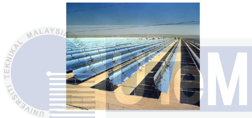
Figure 2.3: Parabolic Trough solar farm [4]
