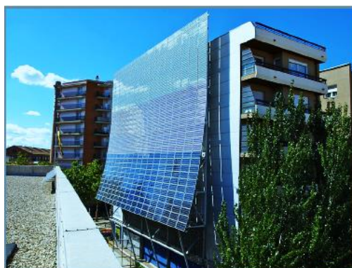
Figure 2.1: Photovoltaic solar panels [5]
