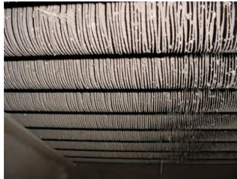
Figure 1.2 Fouling occurred at the outside of the tubes (Tucker, 2012).
