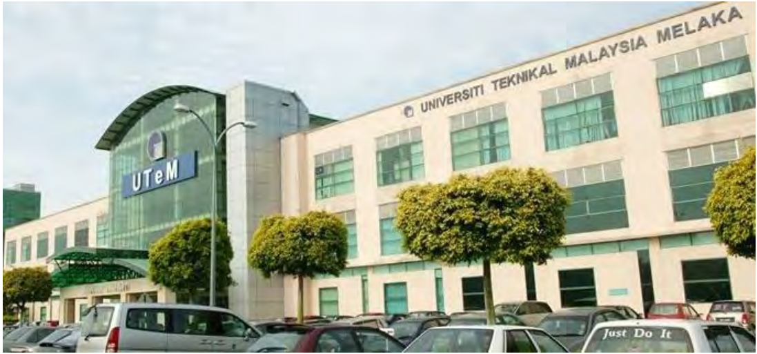
Figure 1.2: Main Building of FTK, UTeM
