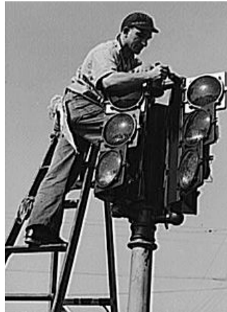
Figure 2.1: The installation of a traffic signal in San Diego in December 1940
