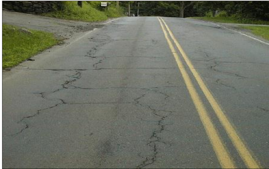
Figure 2.4: Road cracks
