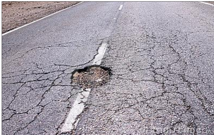
Figure 2.5: Pothole
