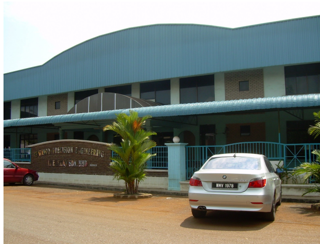
Figure 1.1: Winco Precision Engineering Main Building
