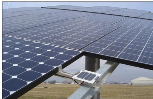
Figure 2.1: Mono-crystalline PV panel
