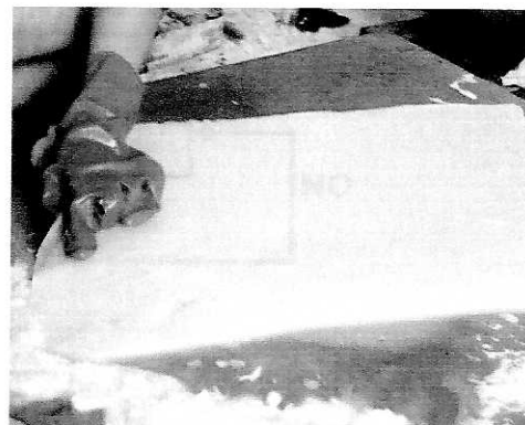
Figure 1.2(d): Finish scrapping
